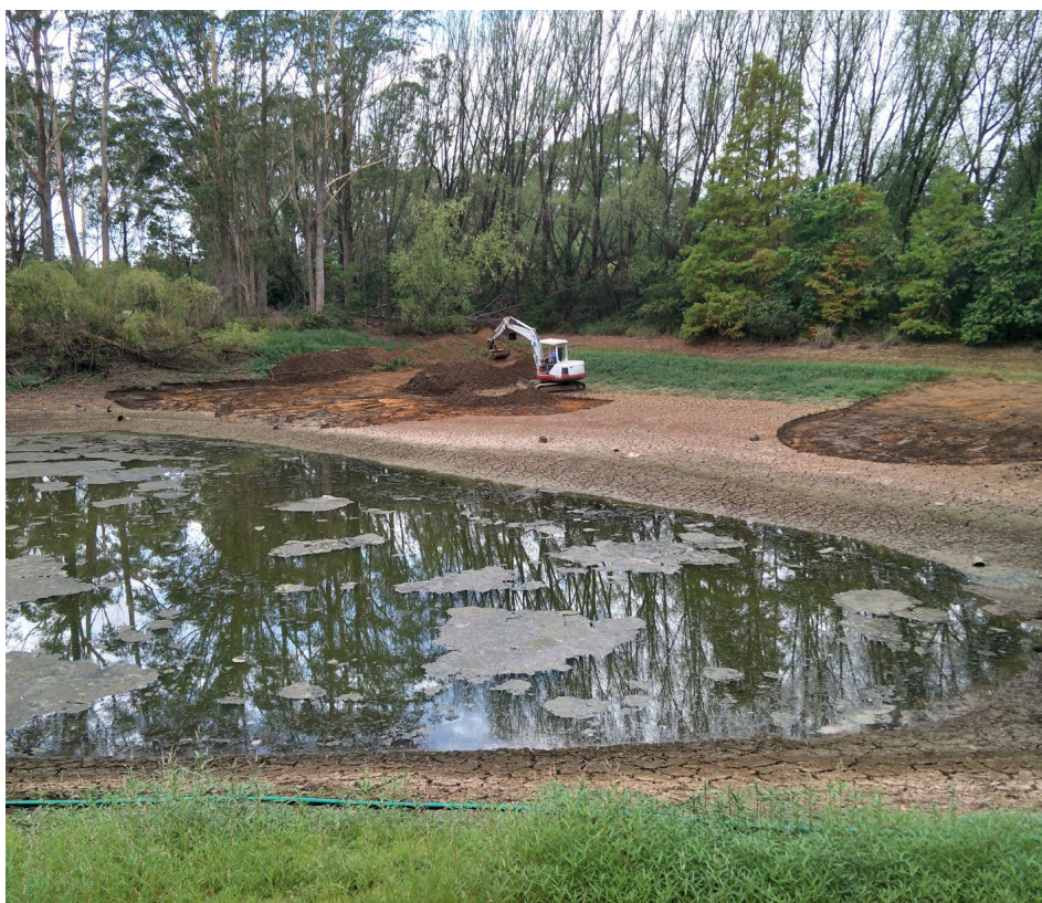
Expanding an existing dam, Engall's Nursery, NSW.
